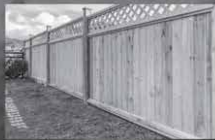
Fence installation: Let us make your property more secure
