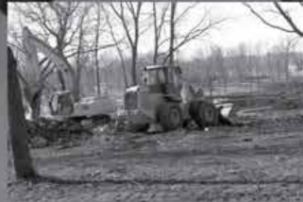
Land clearing: Trust us to make way for your new build
