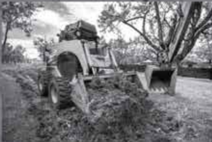
Excavation: Our contractor will prepare your land for any project
